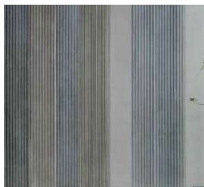
PC PRECAST CONCRETE PANELS WITH FORM-LINER
