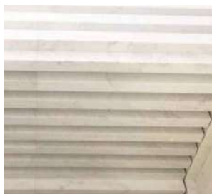
UG CON. SPANDRAL WITH RECESSED GROOVES
